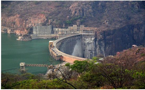
FIG. 7: CAHORA BASSA DAM UPSTREAM VIEW- MOZAMBIQUE
