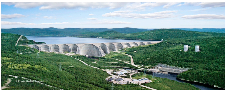
FIG. 6: DANIEL-JOHNSON DAM AND MANIC-5 GENERATING STATION- QUEBEC- CANADA
