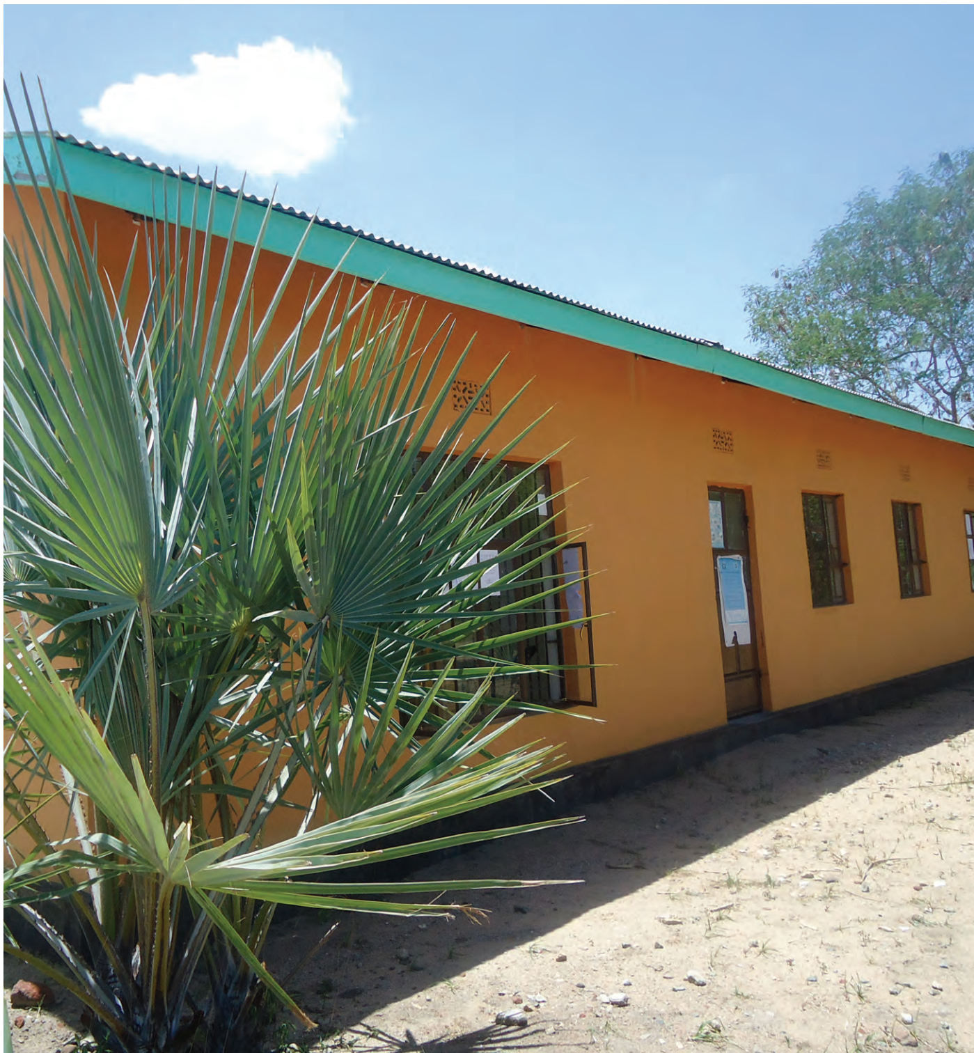
Revenues accrued from WMA, supports development projects like the construction of this village government office.
